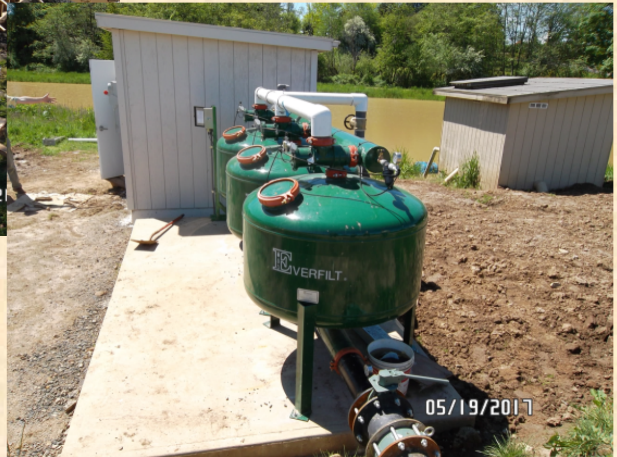
Pumphouse, Flow Meter, sand filtration system is installed
