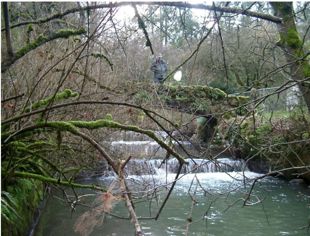
Photo 7. Step Structures on Kelley Creek prior to Restoration
