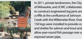
of Milwaukie, and JCWC collaborated to construct engineered log jams and a riffle at the confluence of Johnson Creek with the Willamette River. Over 150 logs were installed to provide cover and shelter for salmon and trout and to allow year-round fish passage over an exposed sewer pipe.
