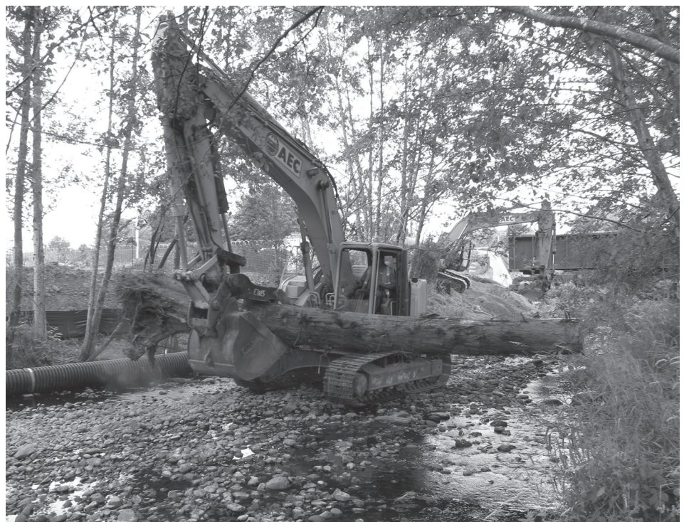
Re-creating channel complexity required major earthmoving equipment to install logs and boulders instream at the Tacoma Street / Johnson Creek MAX station, scheduled to open in 2015.
