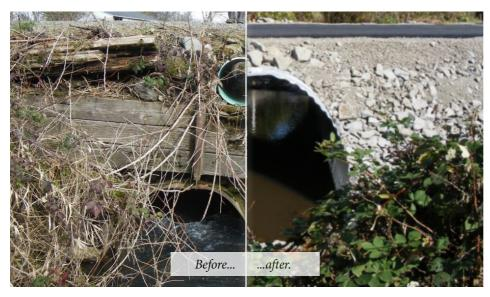
The project was located where Badger Creek passes under the Springwater Trail. The barrier "culvert" under the Trail—actually a set of three rusty and clogged culverts—was replaced with a single, large culvert that should not clog easily. Now fish and wildlife can move freely up and downstream at the site, and can access the 1.6 miles of upstream Badger Creek habitat.
