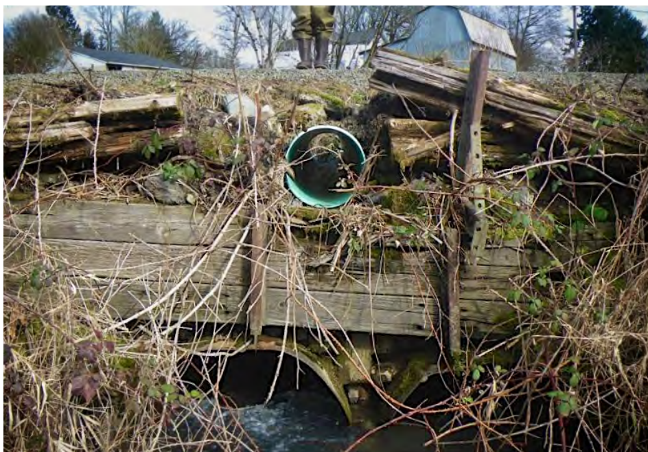
JCWC aims to replace this dilapidated culvert at Badger Creek with a new, fish-friendly one in 2016.
