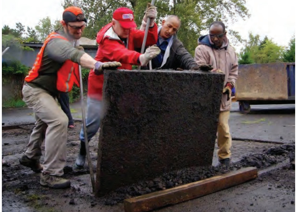
Volunteers came out in force to remove asphalt, condition the soil, and install 500 native plants at St. Mary Ethiopian Orthodox Church this fall.
