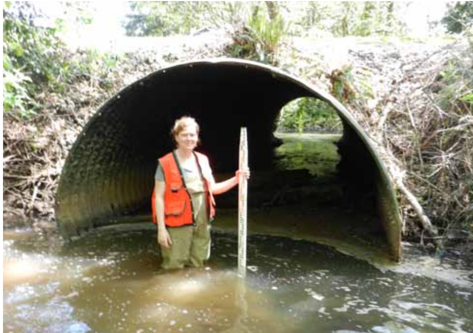
Jan Mehaffy, JCWC fish passage intern, measures a culvert on Sunshine Creek, a tributary to Johnson Creek. Hundreds of culverts are located in the watershed, many of which create barriers for fish passage.
