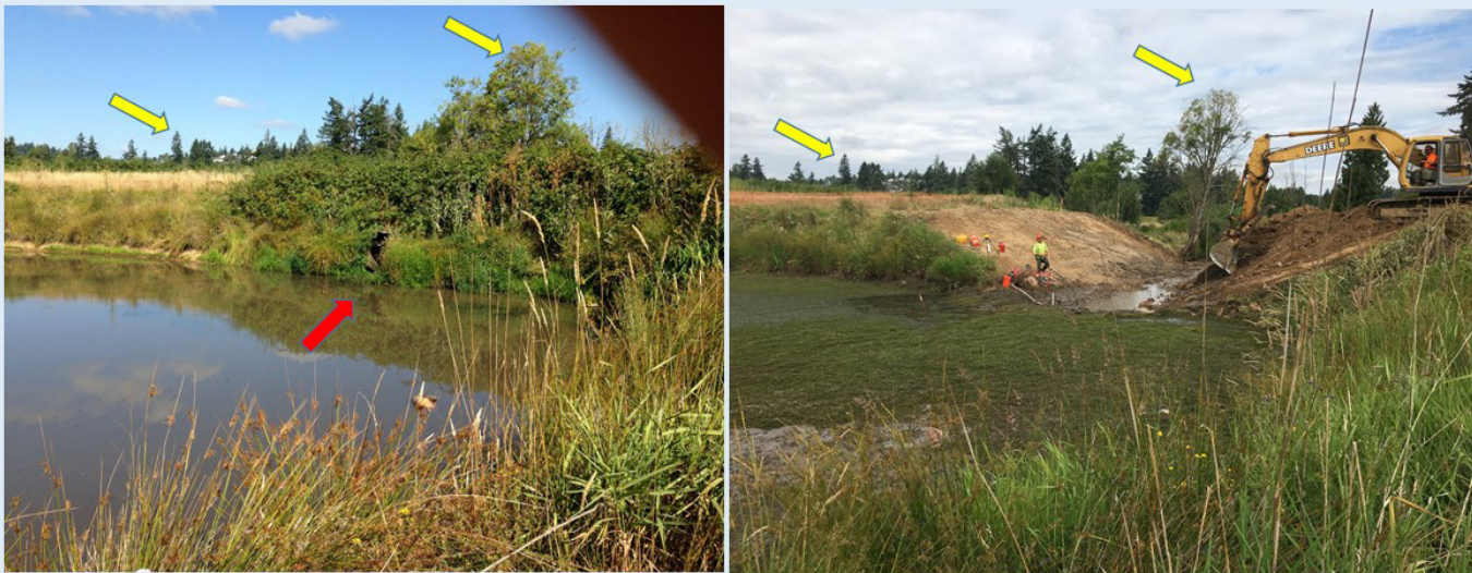
Mitchell Creek / Centennial Pond restoration in progress. Before (l) & Now (r). Yellow arrows identify fixed landscape points for comparison. The old culvert (red arrow) was blocking fish passage and backing up a shallow pond that raised the creek temperature by as much as 14C.
