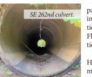
In 2018, JCWC made history when our fish passage project at SE 262nd Street was the first installation in North America of the revolutionary culvert retrofit technology known as Flexi Baffles. This low cost fish passage solution was developed in New Zealand.
