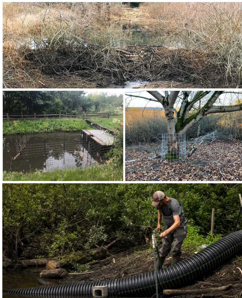
Fig. 3. Beaver dam and beaver coexistence devices in the constructed stormwater wetland facility. Top: main dam near the outlet of the facility as seen during willow leaf-off season. The dam is ~2 m tall and extends along the berms to the right and left for ~100 m. Water can be seen filtering through the dam rather than flowing over it. Middle left: trapezoidal culvert-protector fence. Middle right: tree protection fence. Bottom: pond leveler installed in main dam.
